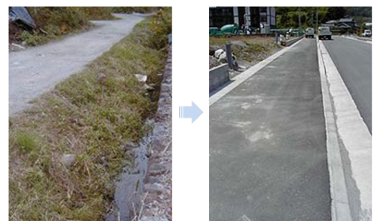
Fig.3 Before and after the land redevelopment project
