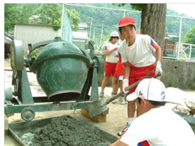
Fig.9 Building the small pool for Medaka
